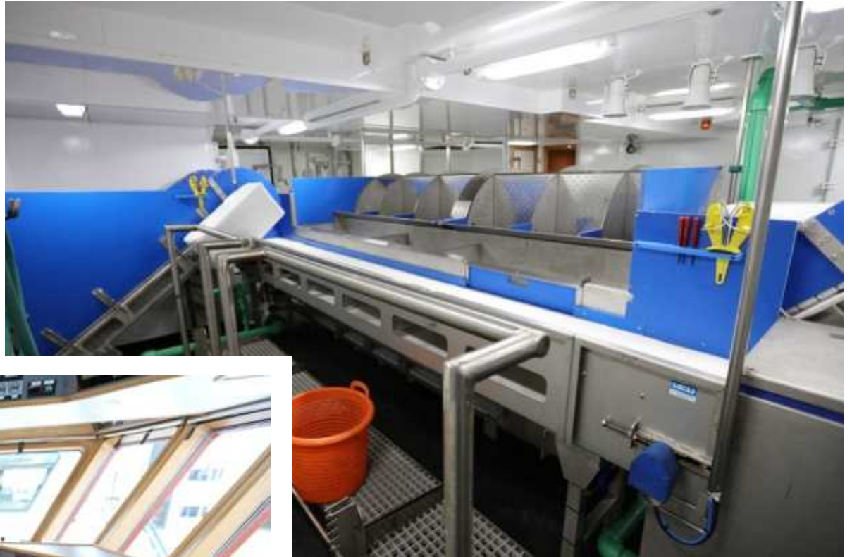
Rosebloom's highly automated fish-handling system is designed to maximise catch quality.
